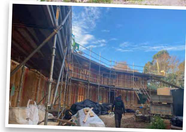
Silvertrees under construction
